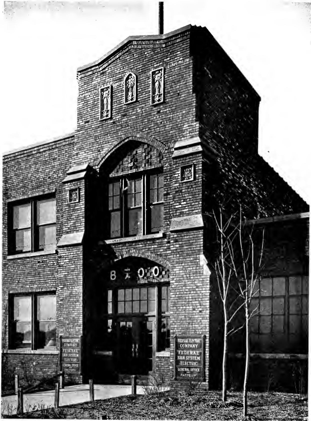
ENTRANCE DETAIL BUILDING FOR FEDERAL ELECTRIC CO., CHICAGO, ILL. GEORGE C. NIMMONS & CO., ARCHITECTS
